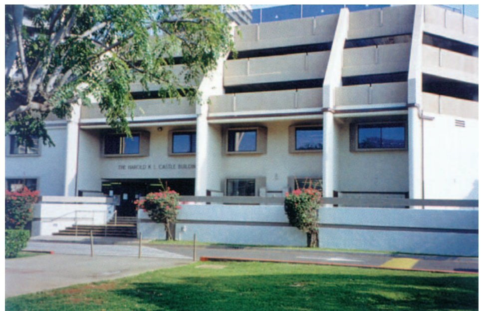
The main building at the Iolani School, Honolulu, where UV lights help control mold and improve the quality of indoor air.
