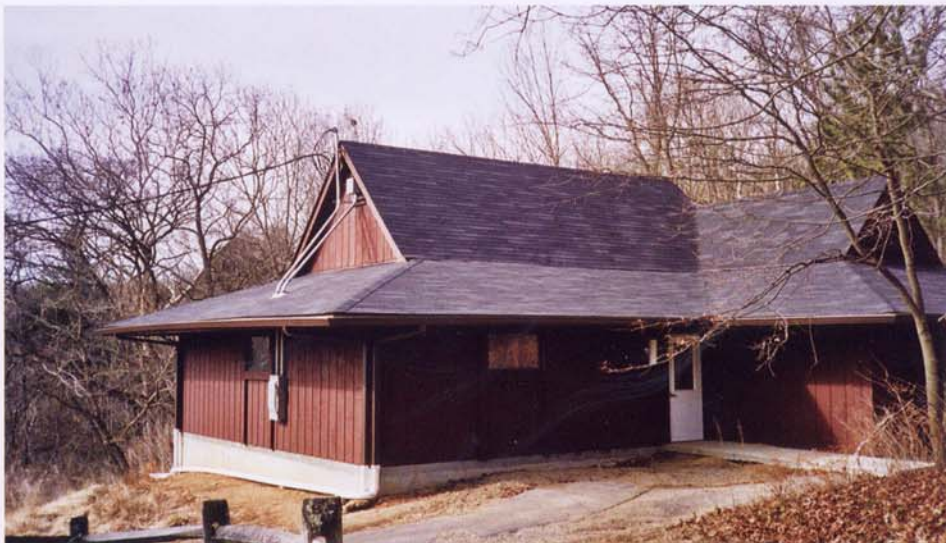
The Stepping Stones Center in Cincinnati faced a problem with mold in the utility room. Pictured is the building after renovation work was completed.
